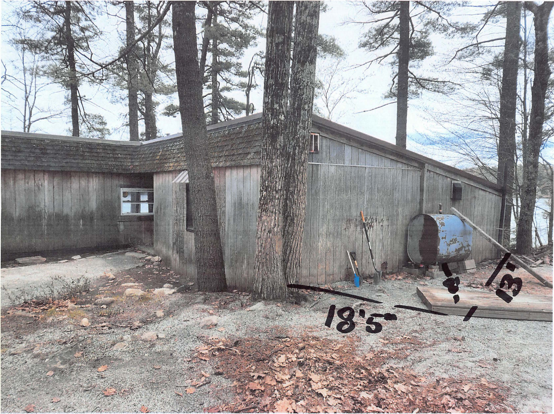
Septic TANK 15 Gile Rd
